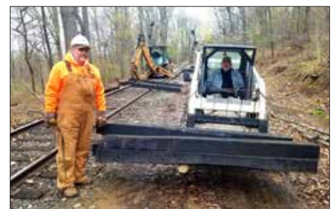
BELOW: Track and ROW Supt. David Kehrer and Jeremy Tuke dropped fresh ties for Scott Symans and his crew to insert into the track on April 27.
