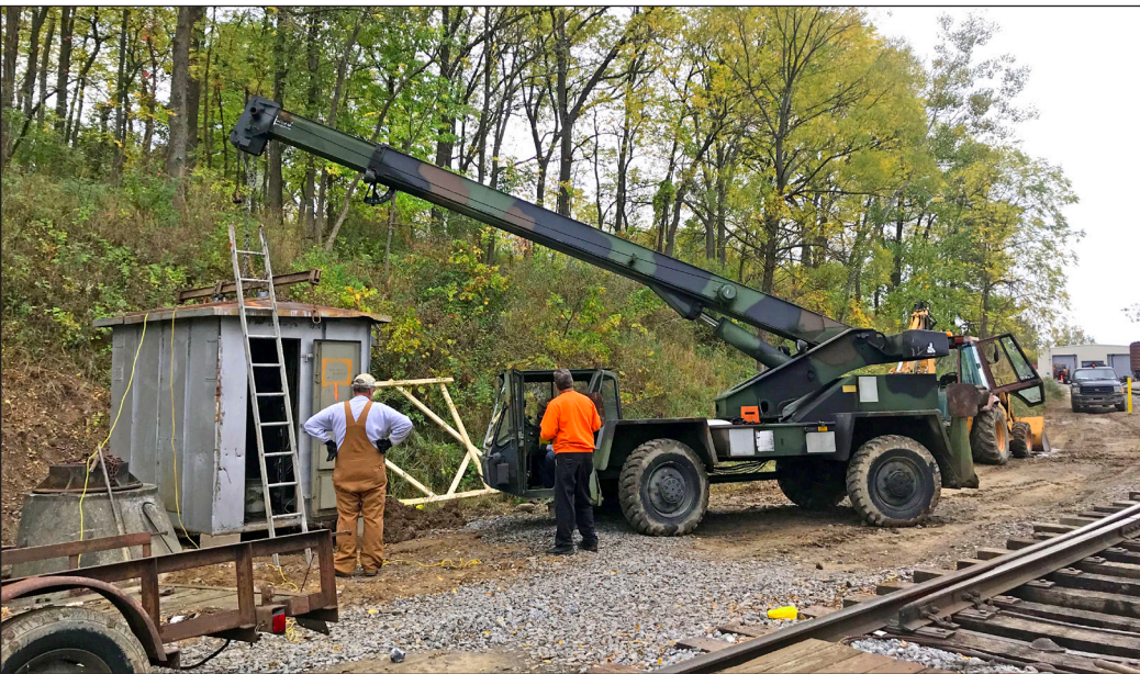
LEFT: On Sunday, October 4, Scott Gleason used our Army crane to lift and position our new signal bungalow onto its foundation at Switch 6. This bungalow housed the relays and circuits that will control the signals around Switch 6 and the Upper Yard.
