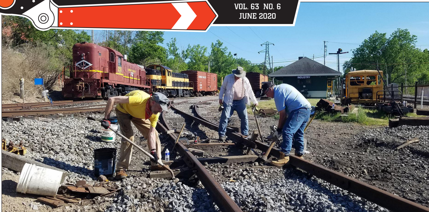
GETTING BACK ON TRACK! The Tuesday Night Track Gang has been tackling the rebuilding of Switch 3 in Industry Yard. Completion of this project will give us a robust and reliable connection to the outside world once again. See page 6 for details. PHOTO BY OTTO M. VONDRAK
