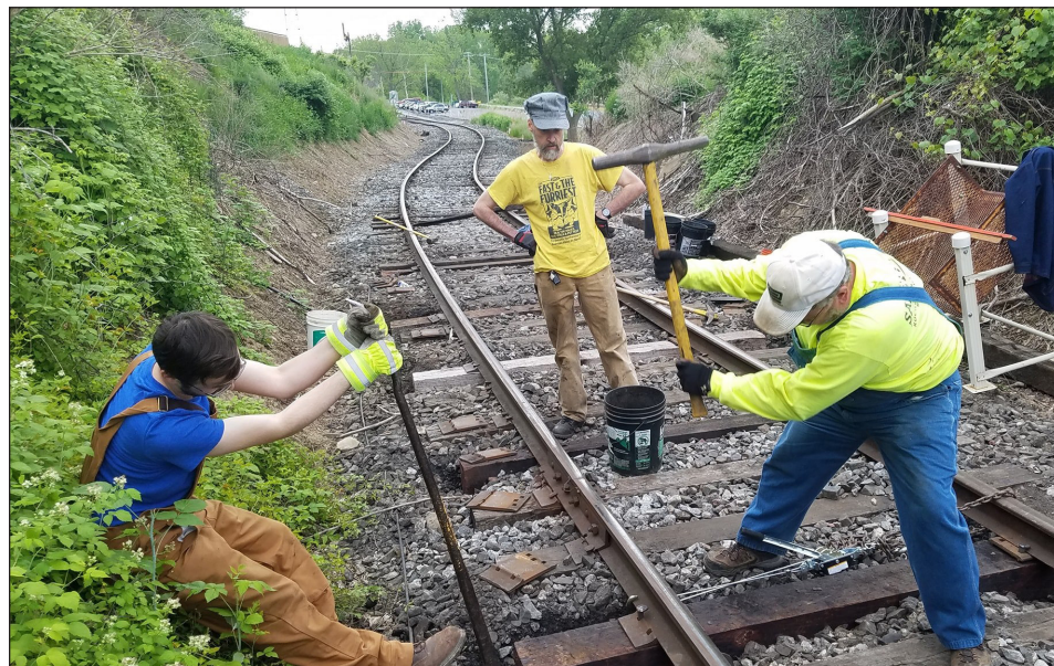
The Tuesday Night Track Gang has been busy replacing ties in the Hill Block through the month of June. Work will continue throughout the summer. New volunteers are welcome!
