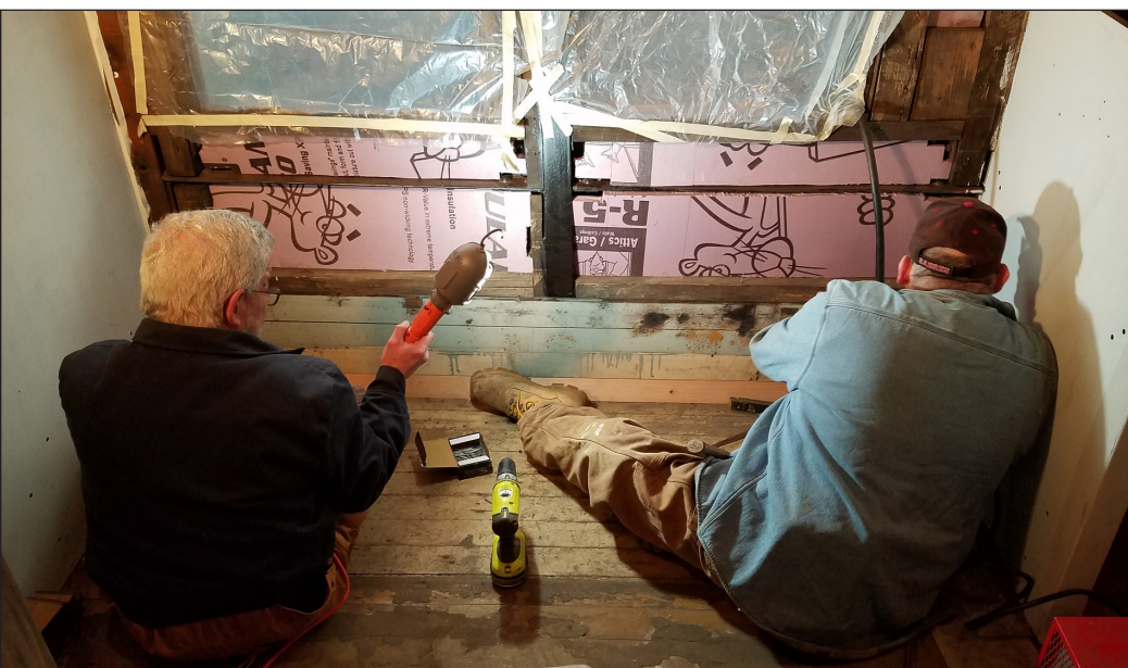
PUTTING THE PIECES BACK TOGETHER: Volunteers Bill Bachmann and Joe Steimer have been busy reassembling the pieces of the northeast wall inside of Lehigh Valley caboose 95100. This caboose was built in 1941 by the LV in their shops in Sayre, Pa., acquired by our museum in 2011.
