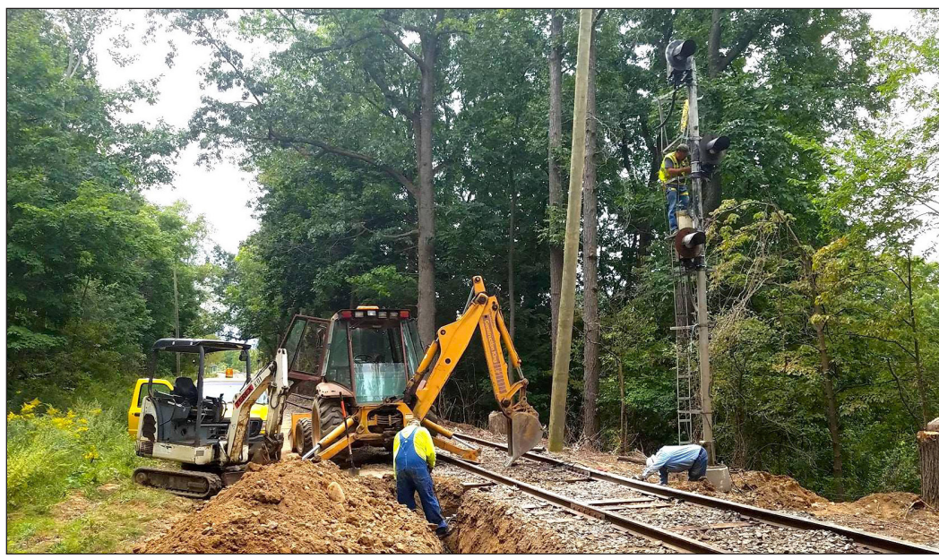
RIGHT: Mike Dow, Dave Kehrer, and Jerry Tusch installed a new block signal at Milepost .3 on September 8. The hardware came from the retired CSX installation at CP 380 in Fairport.
