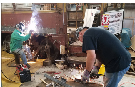
LEFT: Thanks to contractor Crosby-Brownlie, we were able to make a connection with Sheet Metal Workers' Local 46 apprentice program. These volunteers donated their time and skills for professional installation of replacement body panels on Rochester Subway Car 60.
