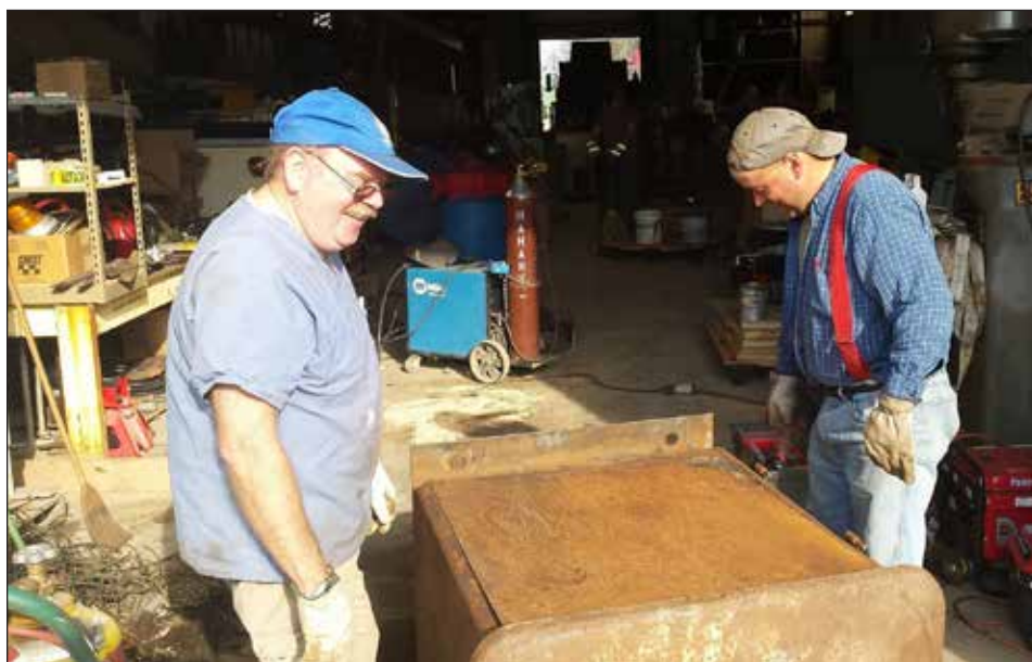
New volunteer Perry Bertsch and museum president Mike Dow weld a new back panel onto an old General Railway Signal cabinet to prepare it for installation along our museum railroad on November 19, 2016. Several projects were completed that will help with infrastructure improvement projects this spring. To get involved with signals and communications, contact Mike Dow.
