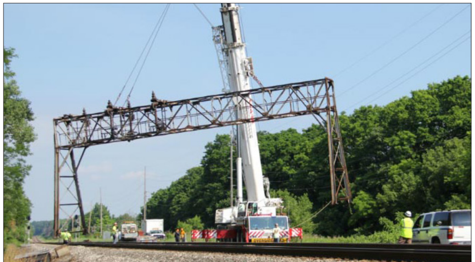
TOP: The New York Central era signal bridge at milepost 365 was casting strong, colorful beams into the night sky on April 11, 2014. Contractors lifted the bridge away from the mainline to prepare for eventual cutting for scrap on June 30, 2014. ADAM LLOYD PHOTOS
