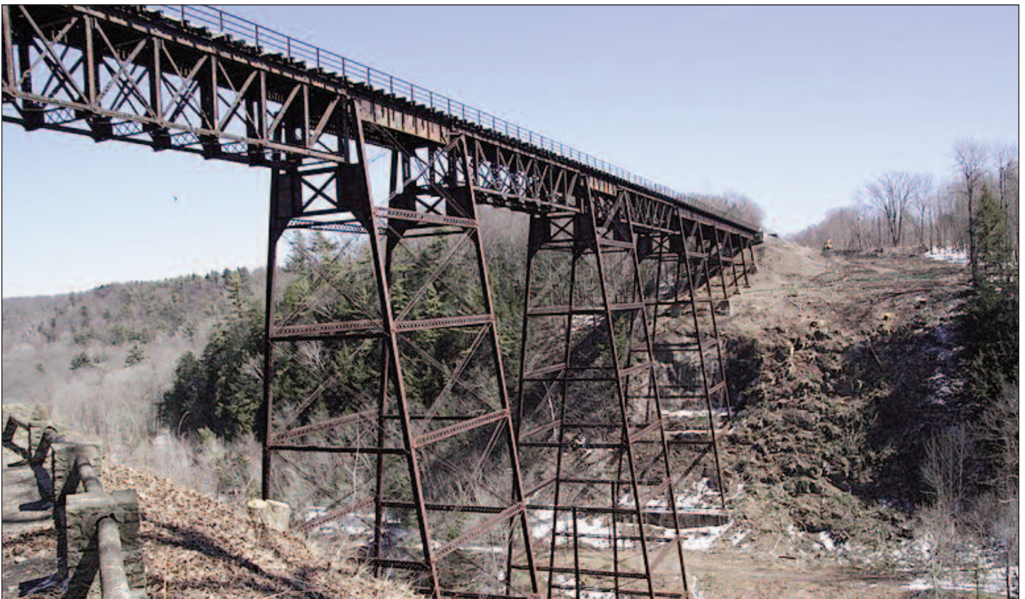
Trees have been cleared as Norfolk Southern prepares to construct a replacement span over the Letchworth Gorge this summer. The trestle dates to 1875, and was built by the Erie Railroad to replace a wooden structure that burned. CHRIS PLAYFORD PHOTO
