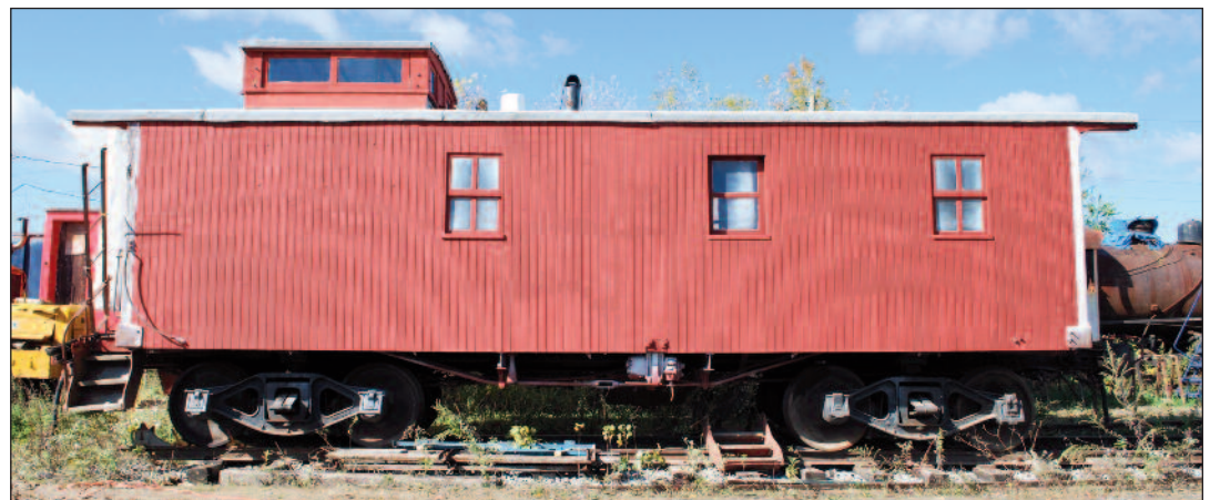
WOODIE WORK: The Marks family has been hard at work on our NYC wooden caboose (1987, built 1921 in NYC's car shop at Oswego). A coat of paint was applied to seal in the new siding, also one king post was replaced. Peter Gores and Chad Timothy worked on the bearing shims to level the car. NYC 1987 poses for its portrait around the end of October, 2010. PHOTO BY JOE NUGENT
