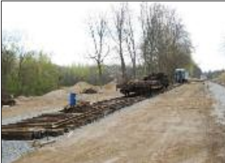
Our new West Siding (ABOVE) was extended by a few hundred feet by our dedicated track department volunteers. As of this writing, the rails have been spiked down and we expect another order of stone to arrive soon. We must move our excursion coaches to this new siding by August. PHOTO BY CHRIS HAUF RG&E 1941 continues to get attention inside the shop (BELOW), preparing for a return to regular service. The unit was successfully started and moved out of the shop in late March and April. PHOTO BY RON AMBERGER
