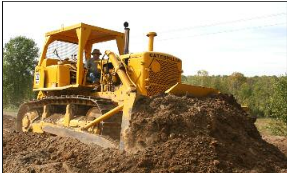
DIG WE MUST: Dale Hartnett checks for subgrade as Scott Gleason waits on the museum's Bucyrus-Erie 20-H hydraulic excavator. Scott was using the 20-H to box out and set the grade at the east side of the excavation for the second phase of the LA&L siding. ABOVE: Dan Waterstraat has the controls of the R&GVRRM's Caterpillar D7E as he starts the excavation for the second phase of the installation of the siding west of the LA&L. PHOTOS BY CHRIS HAUF
