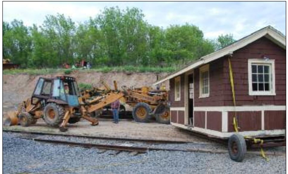
RELOCATING THE RL&B WAITING ROOM: With volunteer Chad Timothy at the controls of our newly donated backhoe, the waiting room negotiates a tight turn in front of the restoration building. The trailer is integral to the waiting room, constructed by the late George Knabb many years ago when the structure was first rescued and brought to our museum. PHOTO BY DAVID SCHEIDERICH
