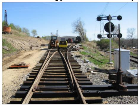
Switch #7! After the first three days of work, switch #7 is constructed and siding #6 (diverging track to the right) is reconnected. The start of switch #8 which will feed the two tracks to the Restoration Building will start just where the front loader is parked.
