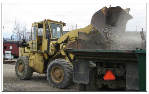
With some better Spring weather and drying ground, it was time to get back to constructing the railroad yard to support the R&GV Railroad Museum's Restoration Building. With 60 tons of ballast delivered to the parking lot of the Industry depot, it was time to load up the ballast for use at the building site. Here the museum's Trojan front loader fills one of the museum's ex-military 5-ton 6x6 dump trucks which will transport the ballast to the work site. [Chris Hauf photos and captions]
