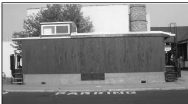
The final product! A white membrane was selected to reflect the sun during summer to assist the air conditioner. (Gale Smith photos)
