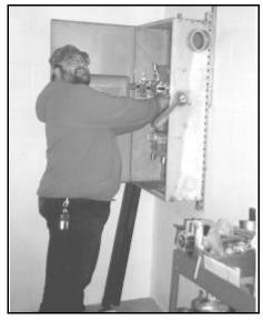
Charles Harshbarger working on installation of electrical components for trolley power substation in the southeast corner of NYMT barn. Our substation team is averaging at least 30 man hours per week on this important priority project. (Rand Warner photo)
