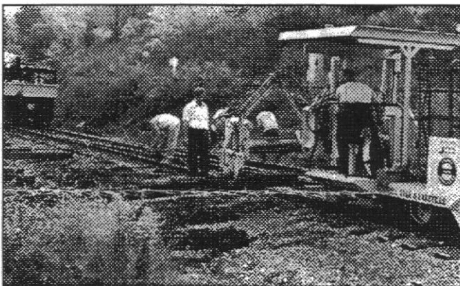
Contractors replacing switch timbers at the R&GV RR Museum yard lead to LA&L main. Interesting to see this tie puller in operation. Gale Smith photo
