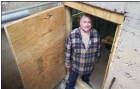
LEFT: Charlie Marks installed a new depot cellar door entrance on November 21. This area was originally the coal delivery chute for the furnace. It was expanded with a new stairwell and doorway in the 1980s.
