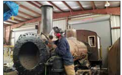
ABOVE RIGHT: On May 23, Bill Marcotte removed the old brackets from Brooklyn Navy Yard 12 that supported an air tank added by the owners later in life. The areas were then ground smooth. The goal is to restore the engine as close as possible to its 1918 as-built appearance.
