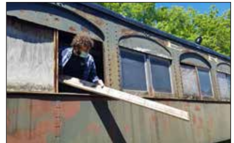
RIGHT: Project manager Charles Rothbart helped remove trash and stored materials as the first step toward restoration of Erie 2328.
