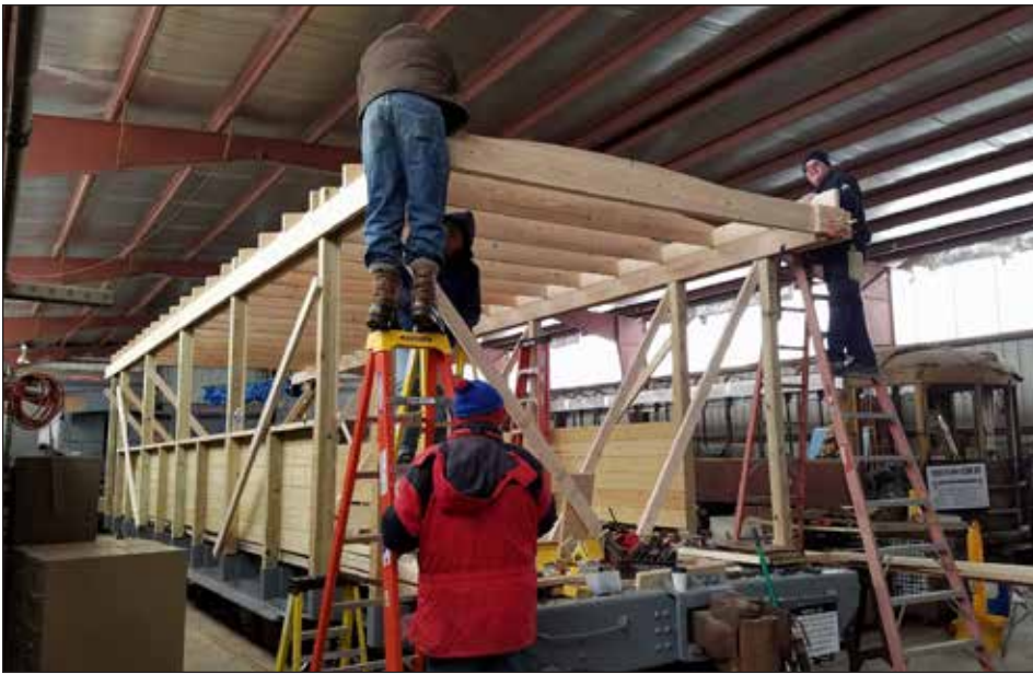
ABOVE: Volunteer Dave Shields assists Perry Bertsch and Rob Burz installing roof rafters on March 4. ABOVE RIGHT: Rob Burz is the project manager on the flatcar project, and is leading the design and construction. We thank Rob for contributing his valuable skills as an independent contractor to this very important project! RIGHT: You can find a “cast of thousands” each Saturday morning contributing to the flatcar project. Volunteers Dave Buckner, Perry Bertch, Rob Burz, Jeremy Tuke, Chris Playford, and Dave Shields were photographed on the morning of February 25 cutting rafters for the roof. Our goal is to place this car into service this summer, to replace the capacity of two cabooses. We will be able to carry more visitors and reduce the number of congestion points for boarding.
