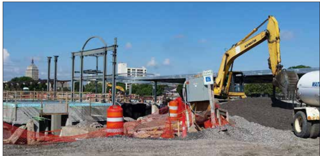
BELOW: Progress continues on the new Amtrak station being constructed in Rochester. New steel has gone up, and work continues on the platform and track arrangements. Two new control points with crossovers have been installed on either side of the new station, which will give the CSX dispatcher greater flexibility in moving freight trains around stopped passenger trains. The new station is expected to open in the fall of 2017.
