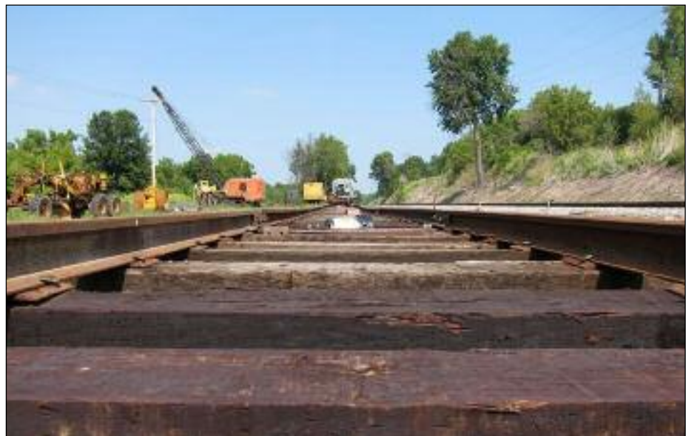
Spikes as far as the eyes can see on September 3! The extension to our passenger car siding has been completed. Now we need to get the ballast deliveries started, but we need your help. Please consider giving to our Donate-A-Ton fundraiser (Online at rgvrrm.org/support). A $20 donation buys a TON of stone and we need at least 150 tons! Please help us continue the progress! CHRIS HAUF PHOTO
