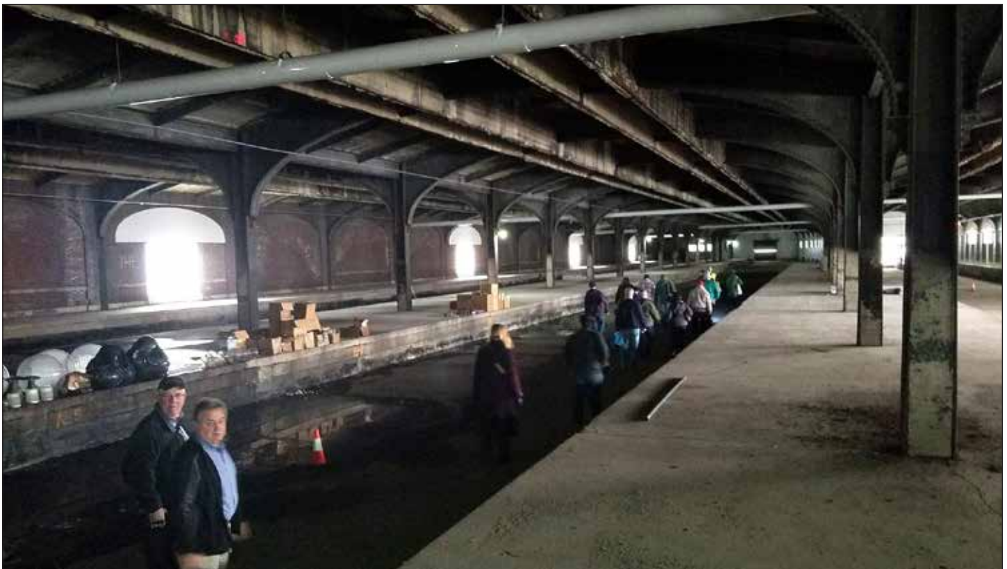
SHUFFLE OFF TO BUFFALO: Museum members enjoyed a private tour of the NFTA Metro Rail shops and yards housed in the old Lacakwanna trainshed in downtown Buffalo on May 6. The upper level passenger platforms were last used in 1962, and the concrete viaducts that ramped up to them were demolished in the 1980s. The troughs were filled with ballast that raised the tracks up to platform level. OTTO VONDRAK PHOTO
