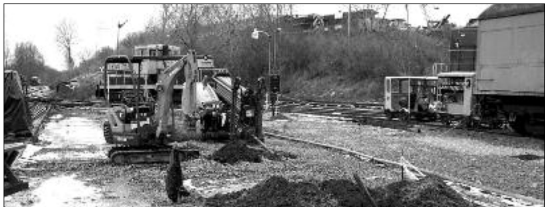
Liberty Underground dug trenches for new water pipes to reach the depot (see page 8). PHOTO BY JEREMY TUKE
