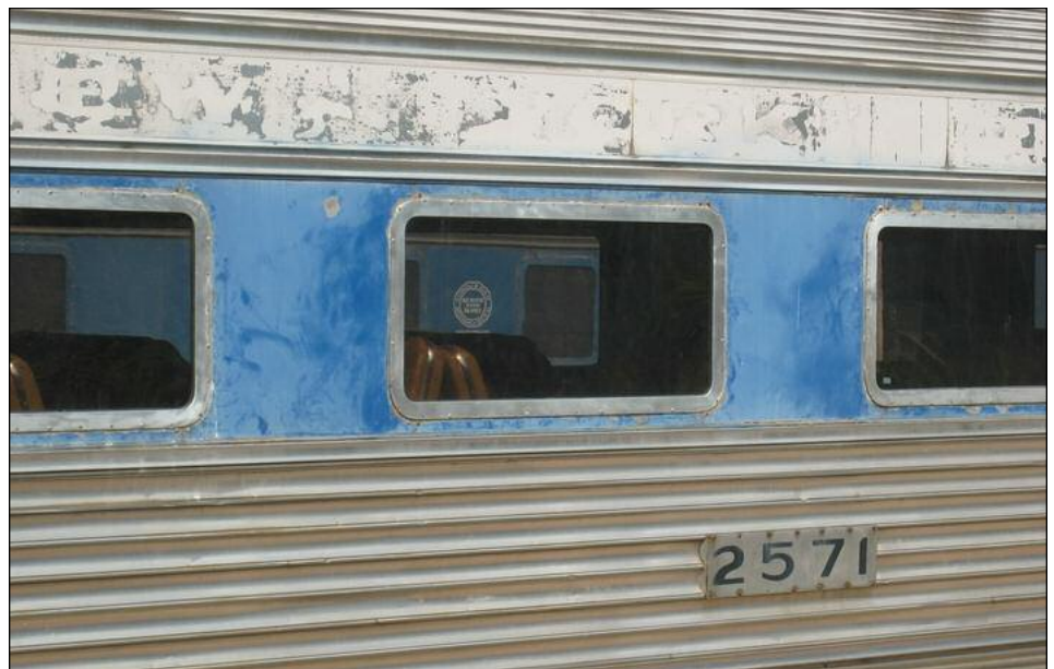
I CAN SEE THE LIGHT: Our coaches now have windows you can see through! The ESE window gang has been hard at work, as evidenced by this photo of 2571. Next up is attacking the blue paint on the window bands, and performing minor interior panel repairs. The removal of all steam heat apparatus continues, with an eye towards electric baseboard heating. PHOTO BY CHRIS HAUF
