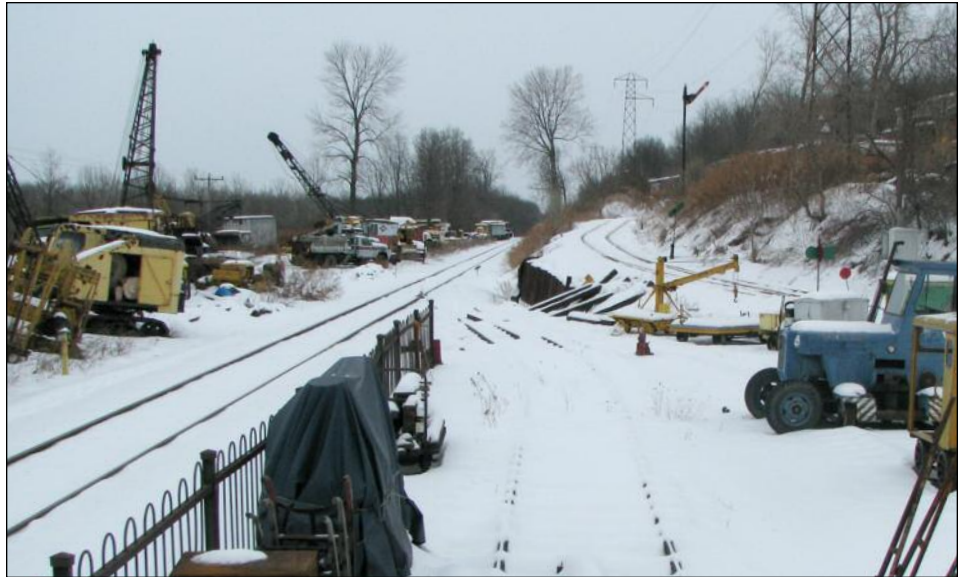
For the first time in more than 25 years, Tracks 1 and 2 at Industry have been vacated. This view is from the top of the steps that once led into the Tool Car (B&O 633). The Tool Car was moved in December and the "Pine Falls" was relocated to the Upper Yard this past summer. PHOTO BY C. HAUF
