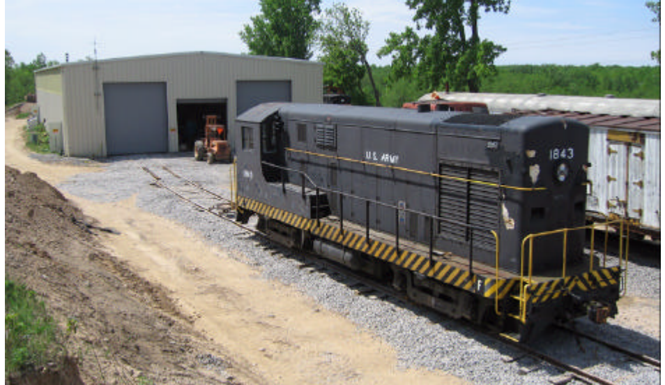
The R&GVRRM's F-M H12-44 #1843 rests on newly built Track #8 in the restoration building yard. As time permits, the dirt bank to the left will be pulled back even further to give the museum even more usable work area around the building. [Chris Hauf photo and caption.]
