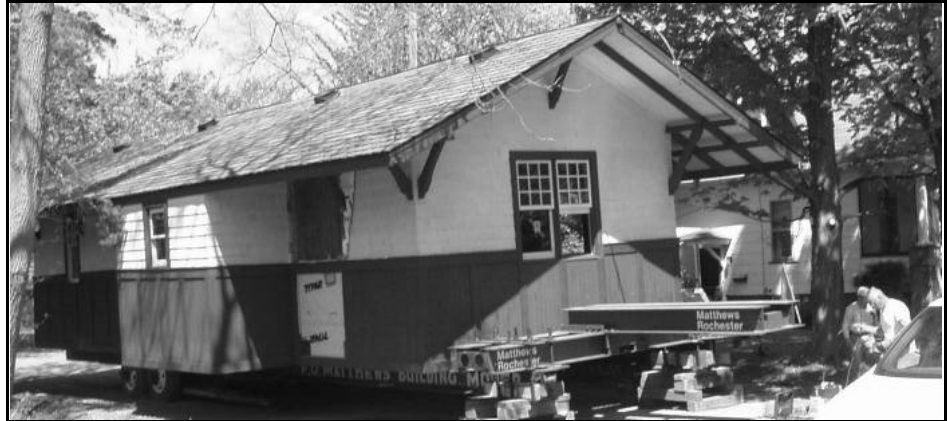
On May 23, the former Spencerport Rochester Lockport and Buffalo interurban depot, freshly painted and with a new roof, sits on a trailer waiting for its grand parade down West Ave. to its new location by the Erie Canal near where it originally resided. It looks great and Bernie Cubitt and crew should feel real proud of their work!
