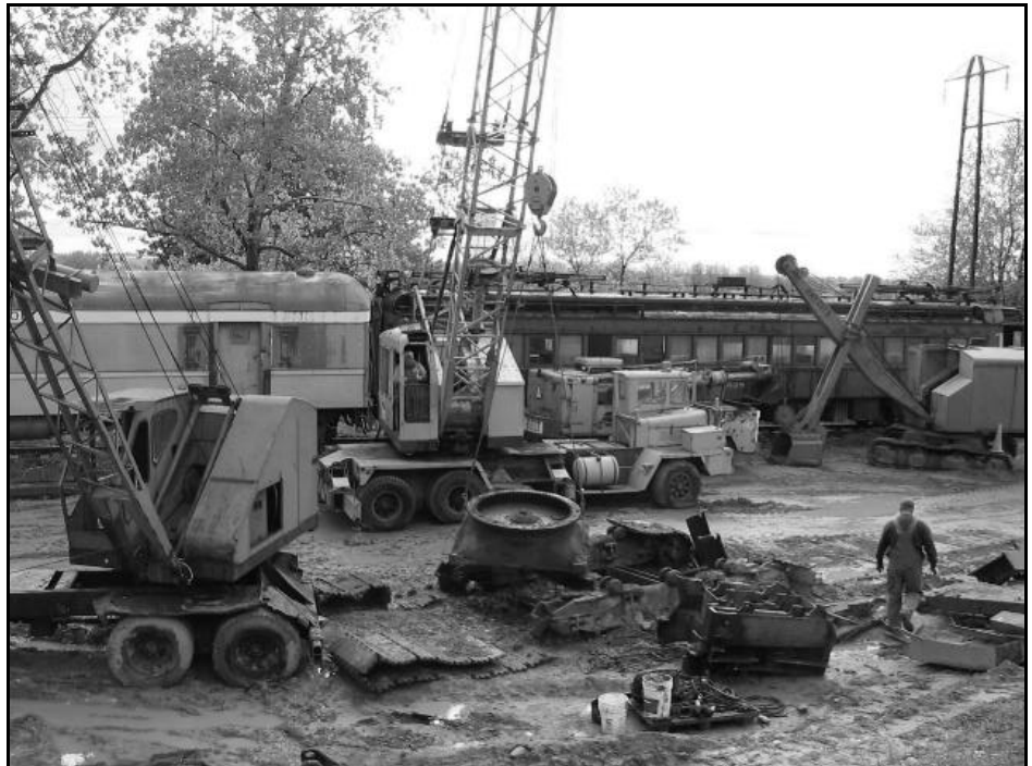
The Northwest 25 crane was used to scrap Koehring 505 excavator on May 24.
