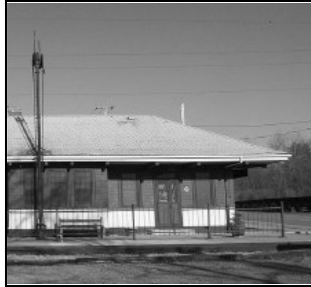
Before the new roof.
