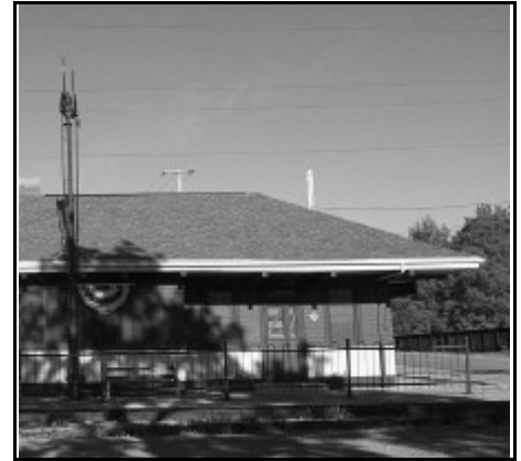
After the new roof!
