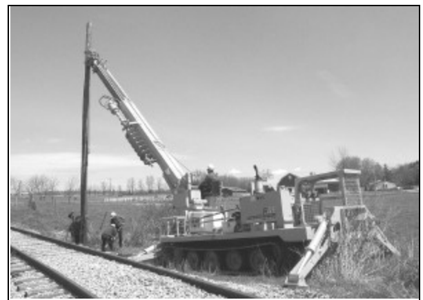
Left, above: Combination crawler crane, auger setting a pole.
